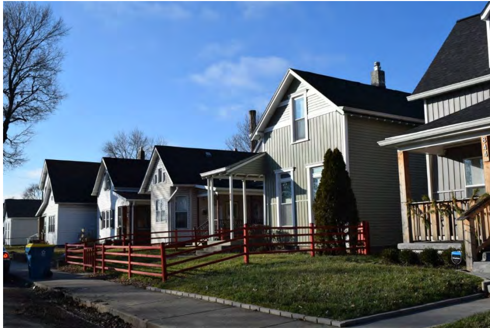
Plate 3. Wright Street within Holy Rosary-Danish Church Historic District, facing southwest.
