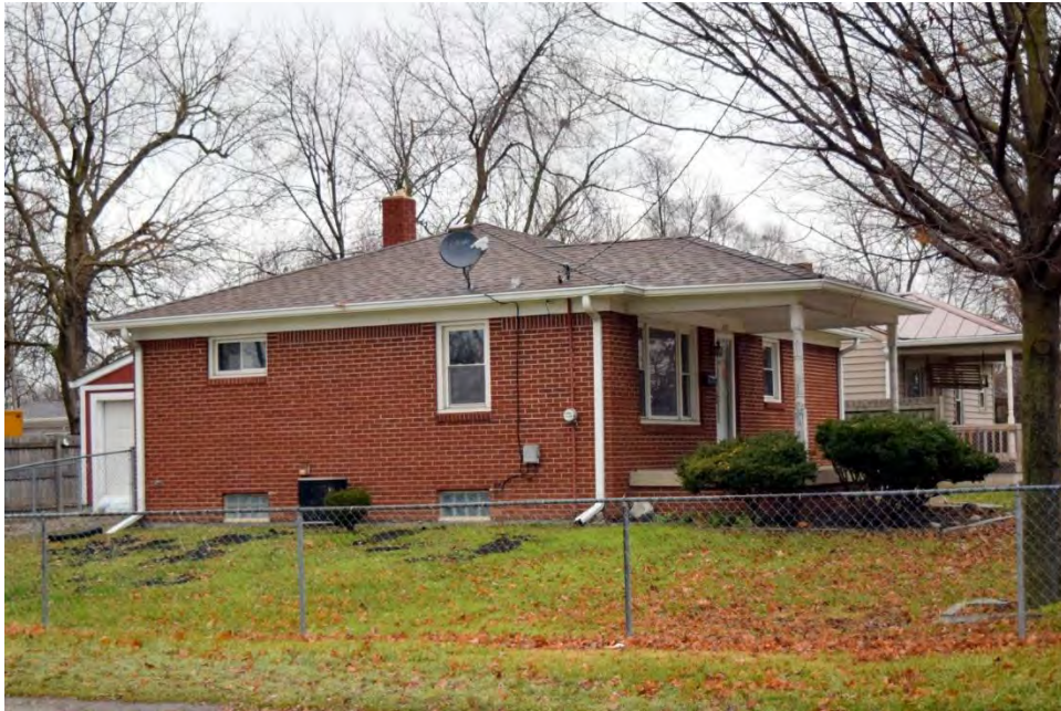
Plate 35. View of a ranch house at 1610 E. Troy Avenue facing northeast.
