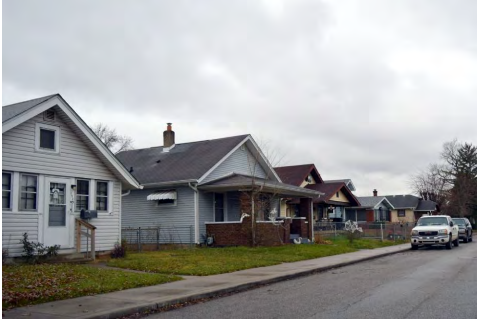
Photo 13. View of the 1200 block of E. Kelly Street, looking northwest.
