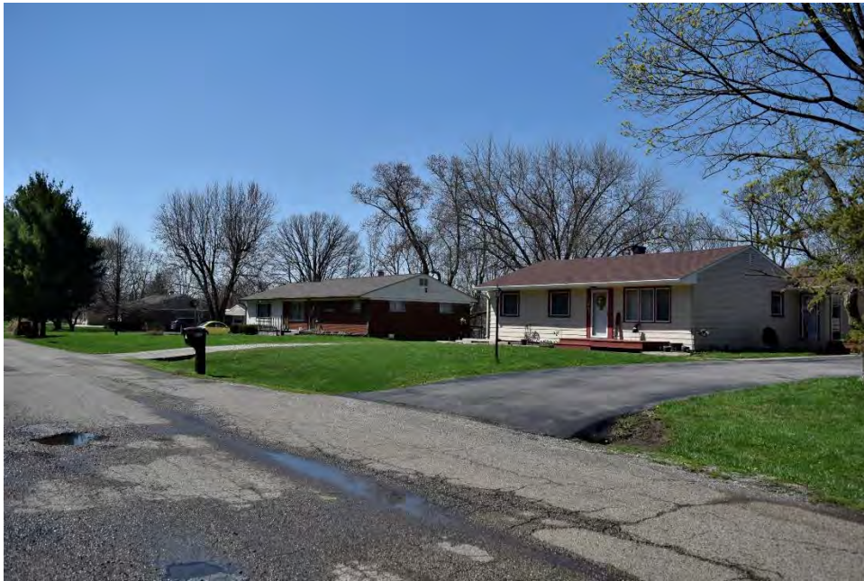
Plate 41. Ranch style homes along South Dearborn Street in the Sherman Drive Park Historic District, looking southwest.
