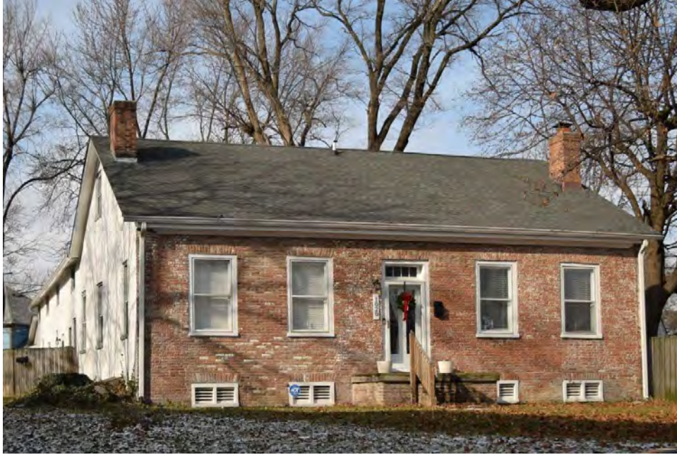
Plate 13. Sanders-Childers House (IHSSI No. 098-296-02550), 1020 E. Palmer Street.
