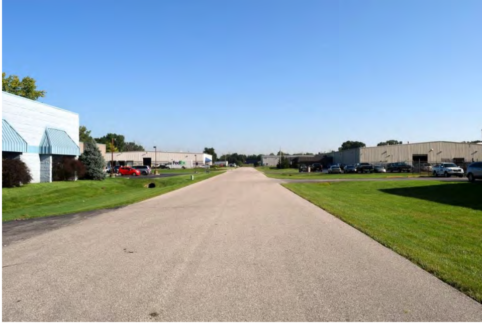
Photo 25. View of Developers Road, looking north toward I-65.
