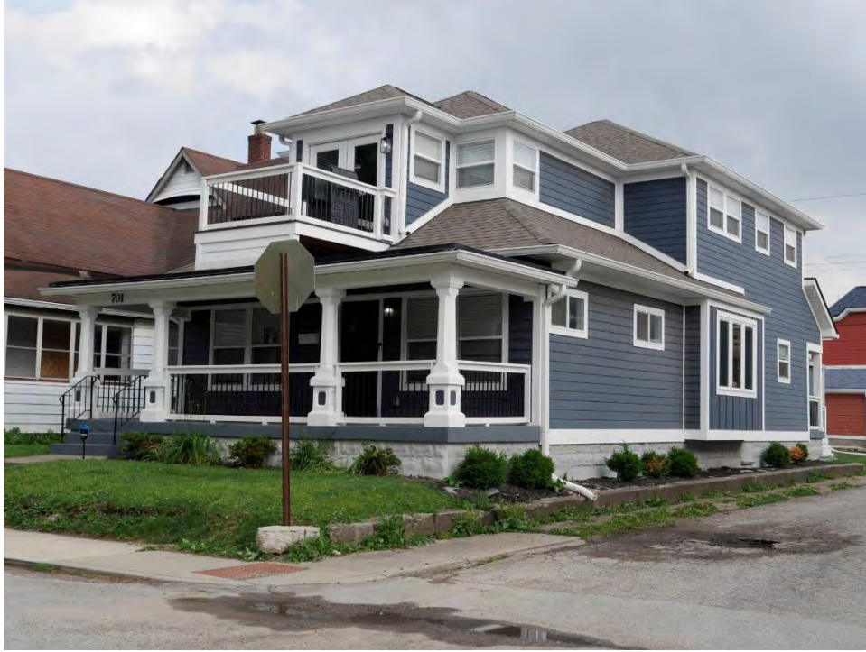
Plate 30. View of the southeast corner of Parkway Avenue and Elmwood Avenue, looking southeast.
