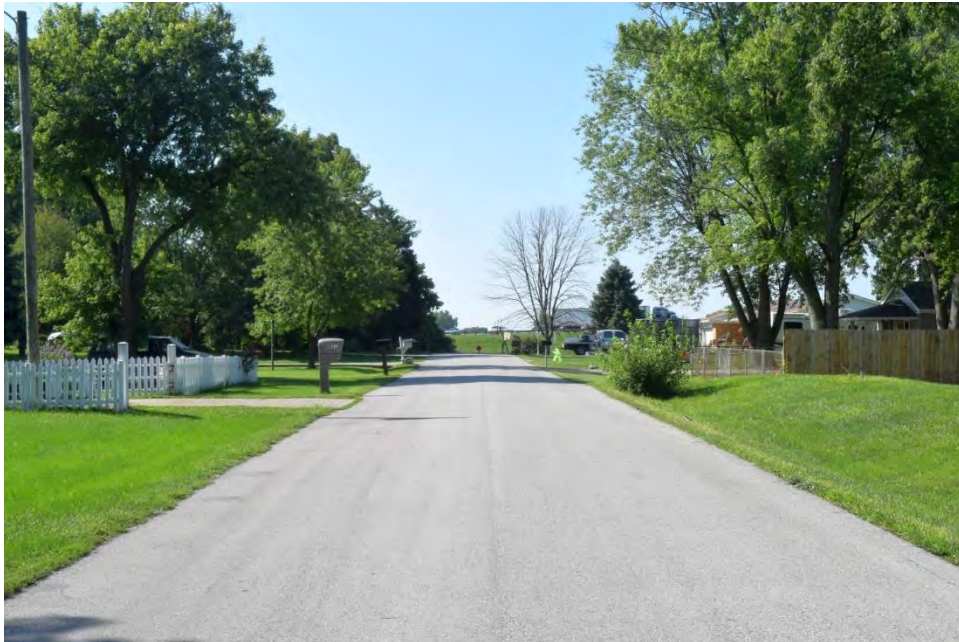
Photo 26. View of S. Tacoma Avenue, looking south toward I-65.
