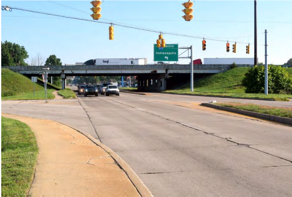
Photo 27. View of I-65 at Keystone Avenue, looking northeast.
