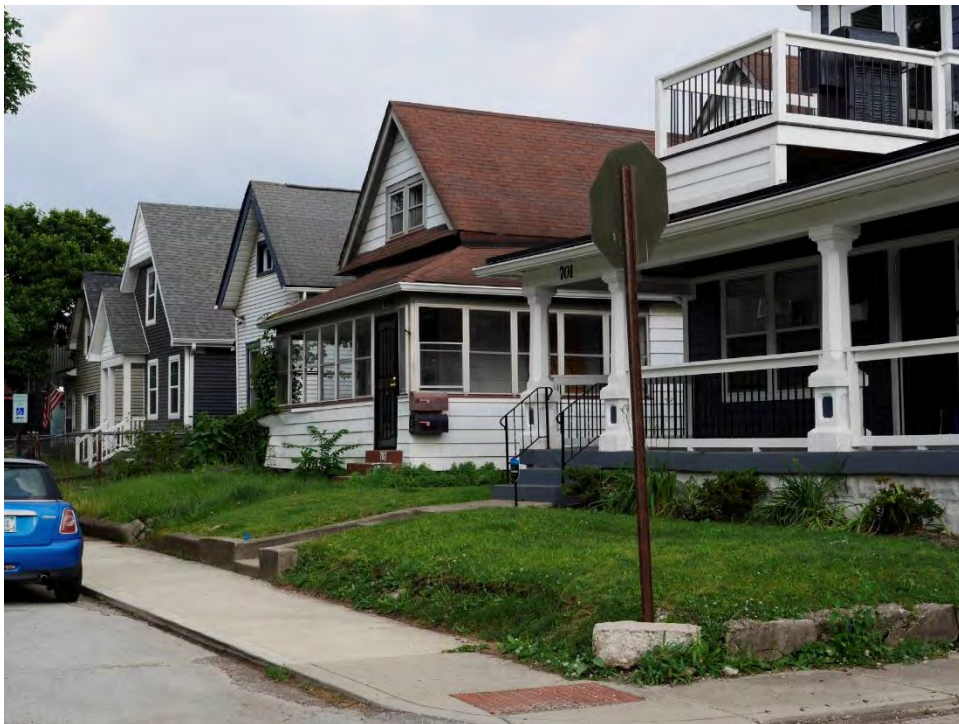
Plate 31. Streetscape view of the south side of Parkway Avenue, looking southeast from Elmwood Avenue.
