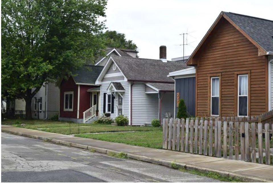
Plate 24. Streetscape view of altered houses at 922–934 Lexington Avenue, facing north.
