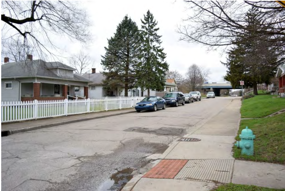
Photo 18. View of E. Southern Avenue at Boyd Avenue, looking west.
