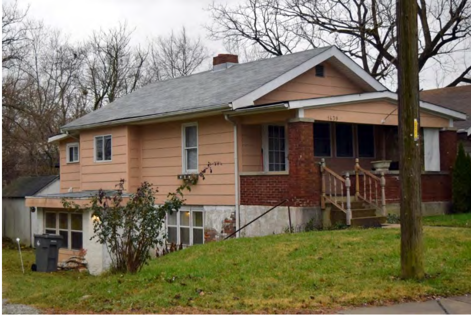
Plate 38. View of 1439 Cruft Avenue, facing northwest.
